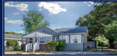
104 W ATLANTIC AVENUE VILLAS, NJ Bayside Beauty
