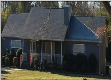
HILLEN Homes - "i>
